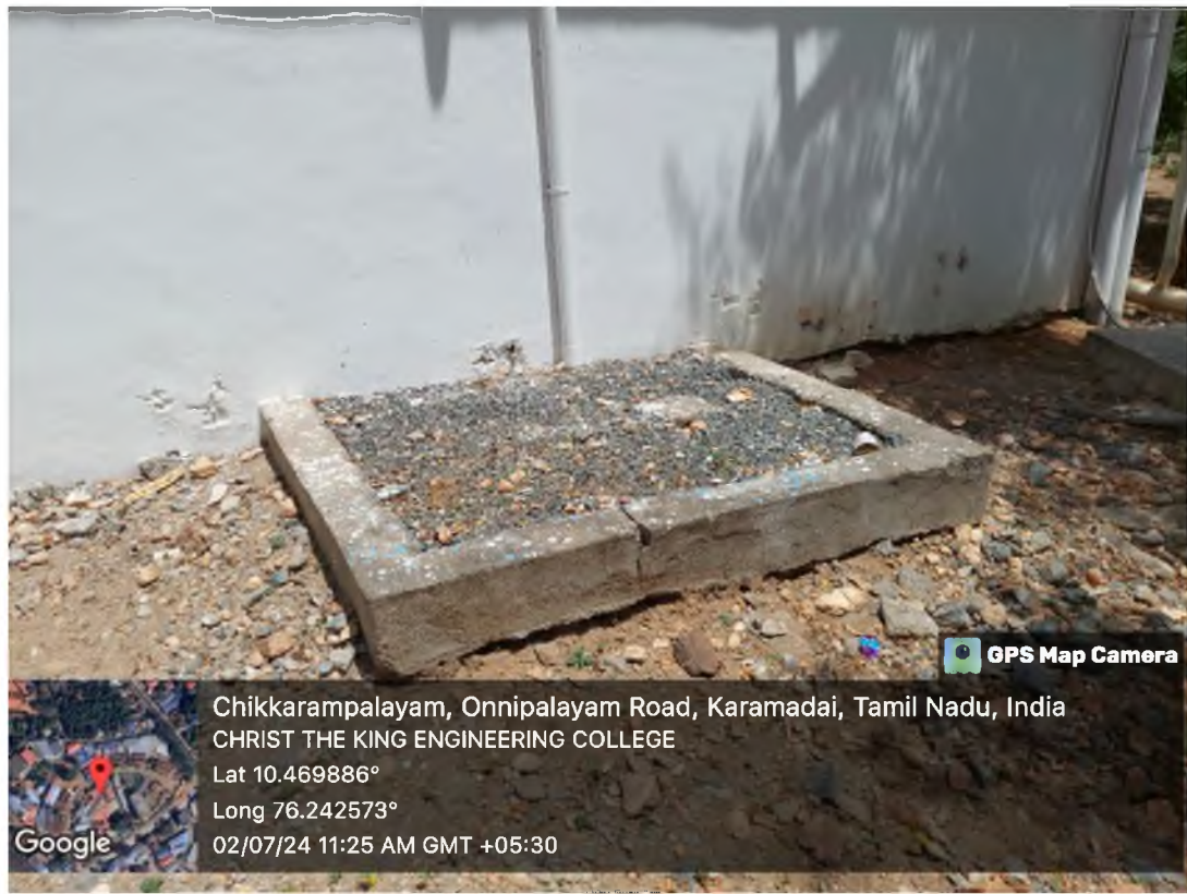
Rain water Harvesting setup outside Mess inside Campus
